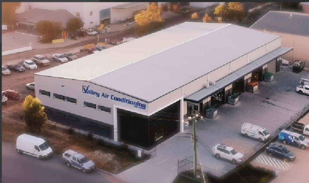
Custom-built Valley Air Conditioning facility.
